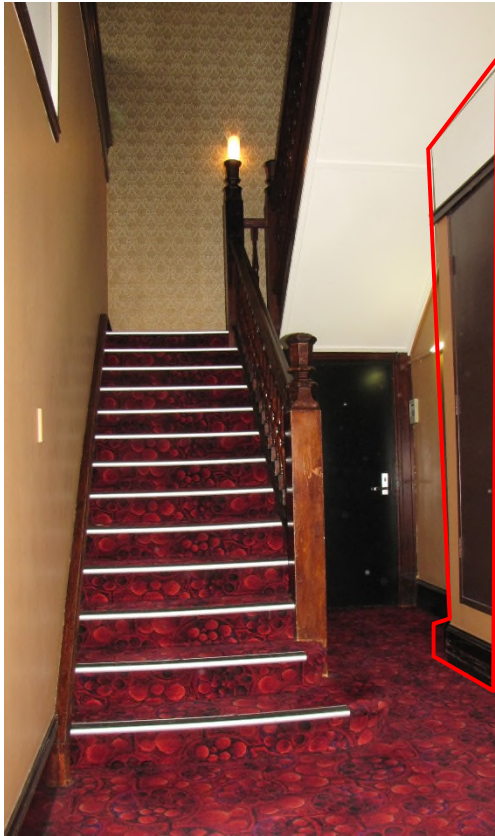
Figure 24: Original Main Stair – from First Floor. Intrusive Main Electrical Switchboard to be removed and original cornice repaired.
