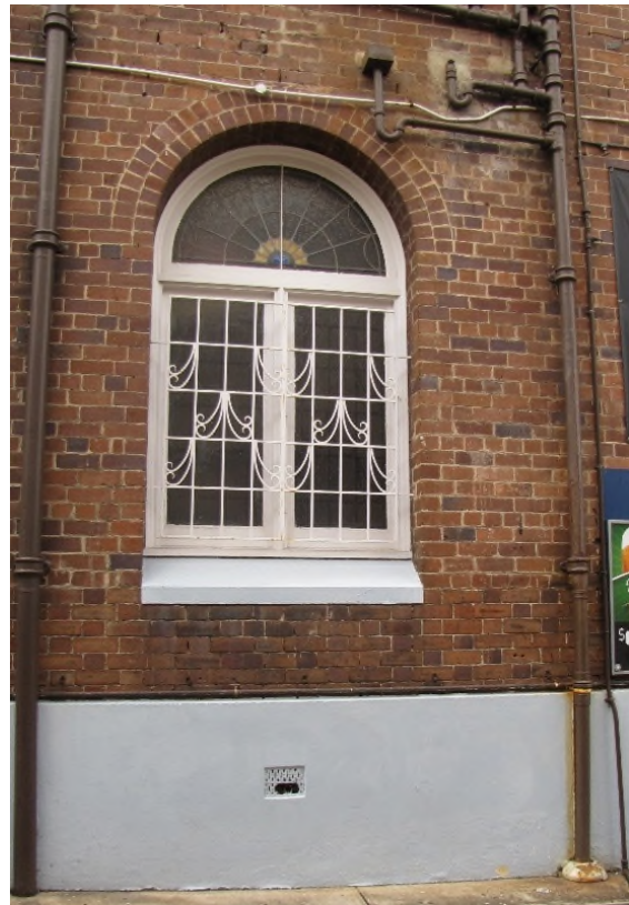
Figure 14: Eastern End Elevation with arched window in face brickwork. Original exposed pipework.
